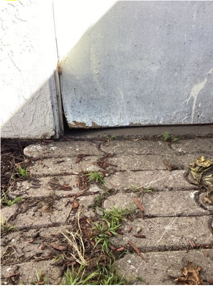
Rear Garage Entry
